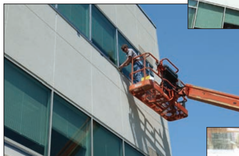
Above: Architectural Testing Forensic Technician prepares the building envelope for evaluation
