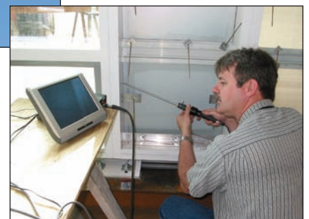
Below: Architectural Testing Forensic Technician Utilizing Boroscope to Identify Leakage
